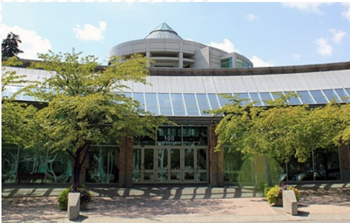
Port Moody Recreation Complex
