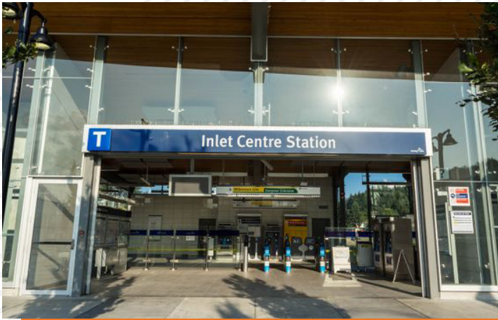
Inlet Centre SkyTrain Station
