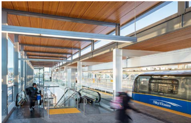
Burquitlam SkyTrain Station
