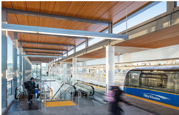
Burquitlam SkyTrain Station
