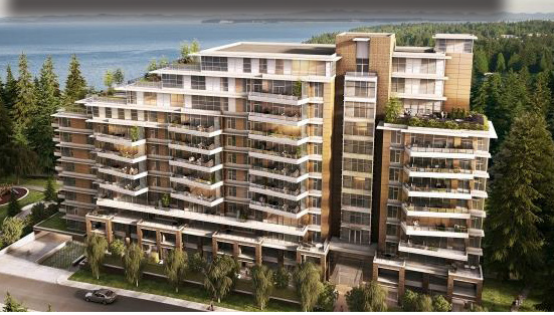
BEVERLY (Under Construction)
